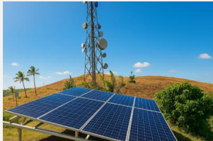
Cell Tower located in Brgy. San Jose (Malabor), Jose Panganiban, Camarines Norte
