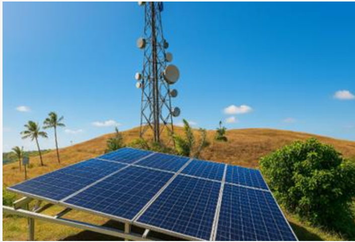
Cell Tower located in Brgy. San Jose (Malabor), Jose Panganiban, Camarines Norte
